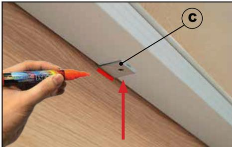
5. Align L-Bracket to the holes underneath the noticeboard and mark the position on the wall.
