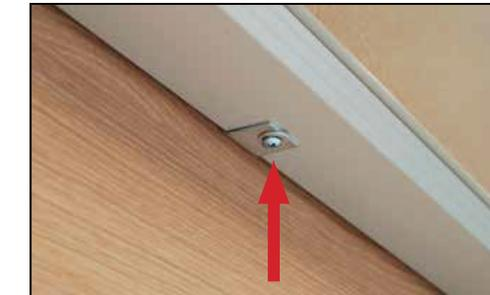
7. Mount the board on the wall and screw the L-Bracket to the board to secure the board on the wall.
