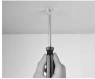
2. Determine the position of the sign and drill a hole for each fitting into the ceiling. Screw the top half of the fitting into the ceiling.
