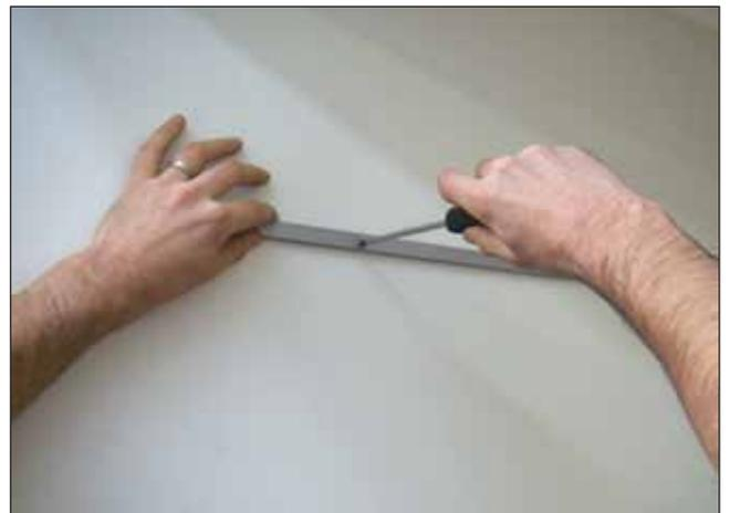
3. Mark the wall with the desired position of the hanging rails. All measurements should be between the upper and lower edges of the rails. The rails must be oriented as illustrated
