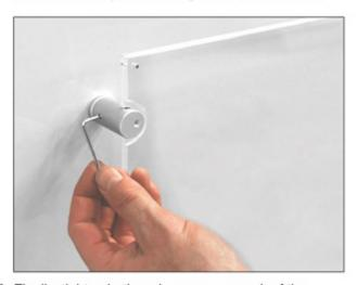
Finally, tighten both grub screws on each of the upper stand-offs to fasten the sign in place
