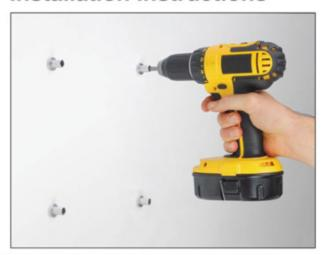
Mark out the position of the stand-offs as per the table above and screw the wall brackets in place using the screws and wall anchors provided
