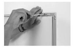
Drill holes and insert the wall anchors into the wall. Set the DY03 in place and screw to wall with the included screws.
