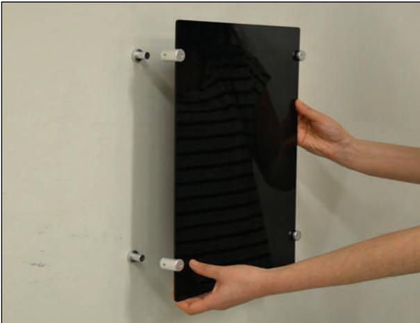
3. Once the upper stand-offs are assembled to the acrylic, slide the assembly onto the wall pieces. Fine tune the position of the upper pieces as required
