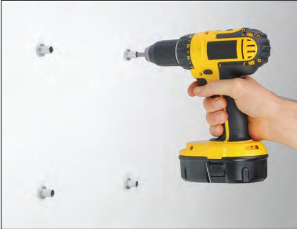
1. Mark out the position of the stand-offs and screw the wall brackets in place using the screws and wall anchors provided
